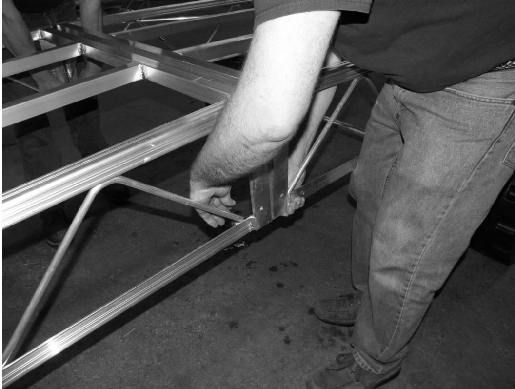
FIG. 32: Install End Platform Section to Assembled Dock Sections
